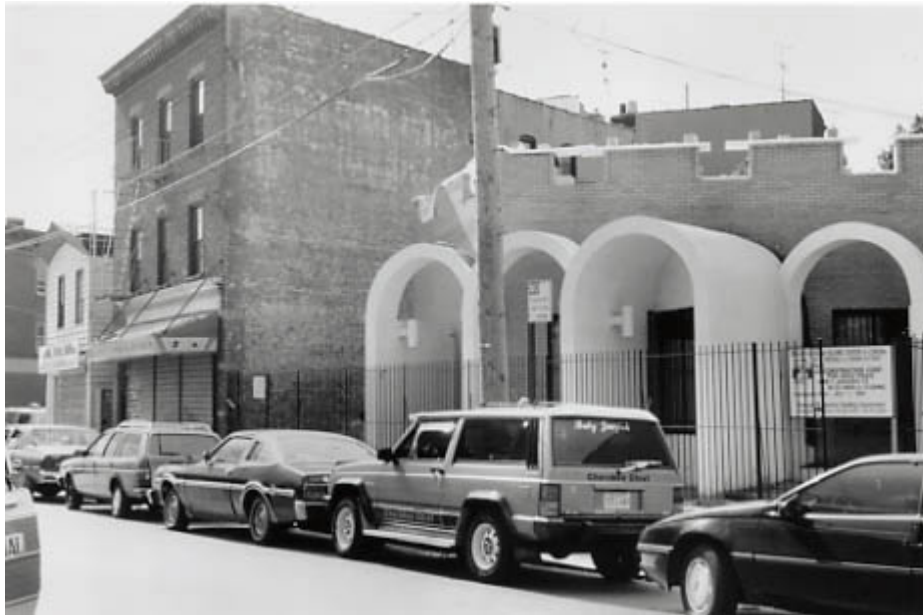
Masjid Al-Falah Hanafi Sunni mosque in Corona, Queens under construction.
